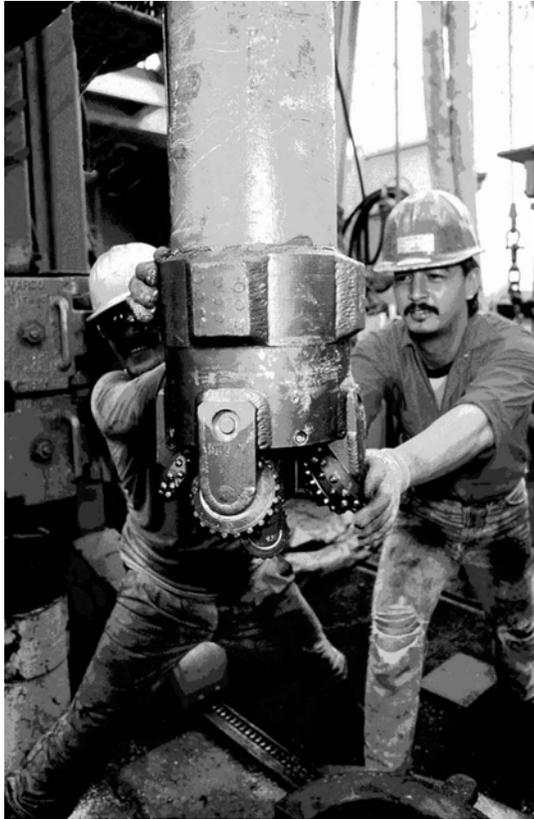
Fig. 14.05. Handling the massive drill collar at the rotary table of the drilling vessel requires skill, brawn and caution.
